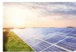
Energy Storage System
